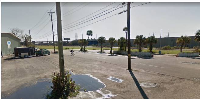
Existing conditions at the intersection of Hackemann Avenue and Meeting Street
