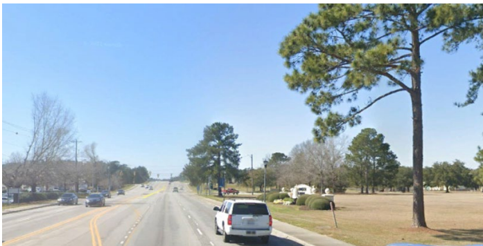
Existing sidewalks along Rivers Avenue (US 78)
